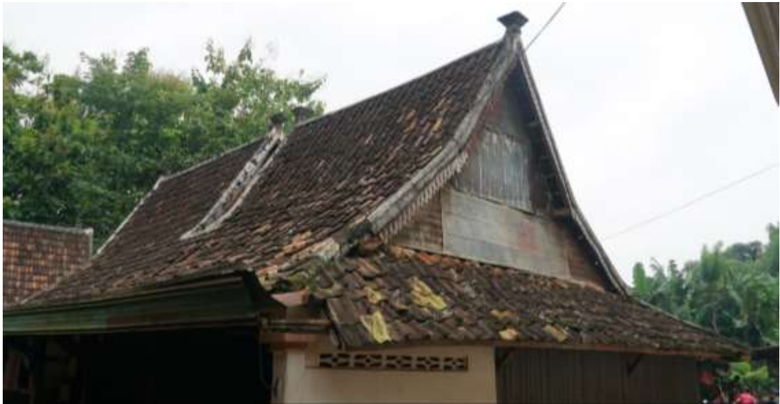
Photo 18: Double-ridged Trompessan roof with a Pacific influence on the roof's crown. Source: Author Document 2023
