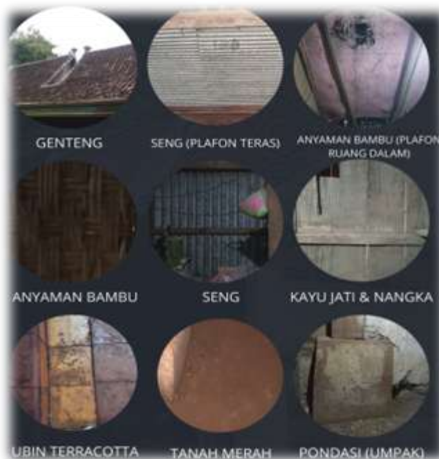
Photo. 09 Top, Roof and Ceiling Materials
