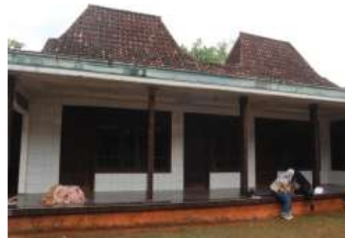
Photo 04 : Taneyan Lanjheng Brick Wall Source: Author Document
