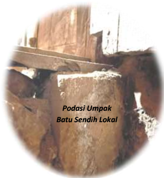
Photo. 7 : Left. Stone foundation using local Sendih stone. Photo. 8 Right. Main pillar/bed pillar using local jackfruit wood. Source: Author Document 2023
