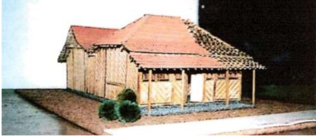
Photo 16: Peghun Roof Shape with Truncated Roof on the Right and Left Sides. Source: Author Document 2023
