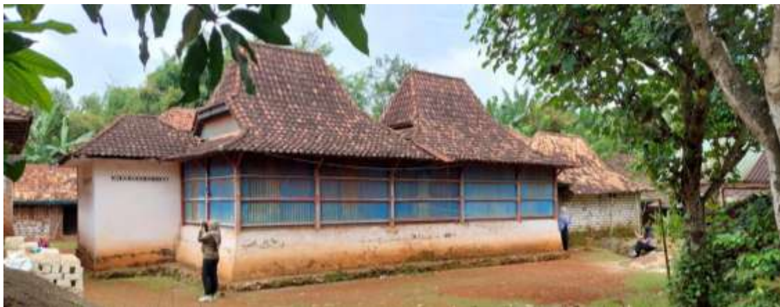
Photo 17: Double-ridged Jhaddhri roof with truncated eaves on the right and left sides. Source: Author Document 2023
