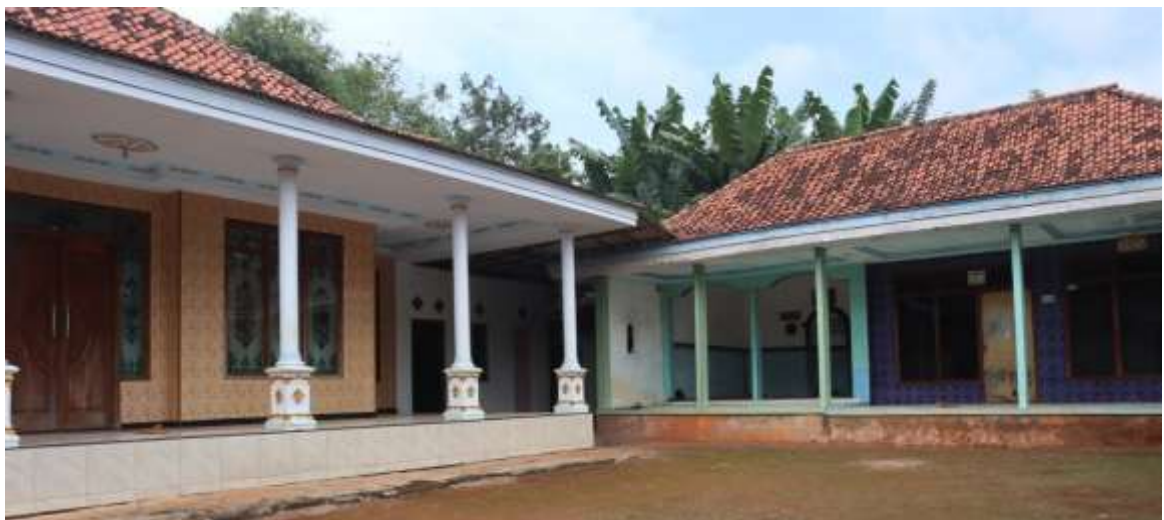
Photo 19: Contemporary Roof Design Using a Shield-Shaped Roof and Tile Roof Covering Source: Author Document 2023
