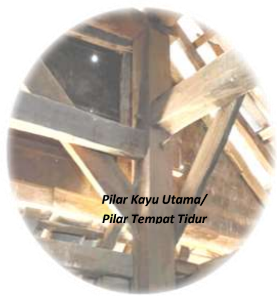
Photo. 7 : Left. Stone foundation using local Sendih stone. Photo. 8 Right. Main pillar/bed pillar using local jackfruit wood. Source: Author Document 2023
